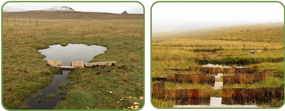
Figure 3. (a) Blockage at the outlet of a pool and (b) Blockage in a drainage system.
